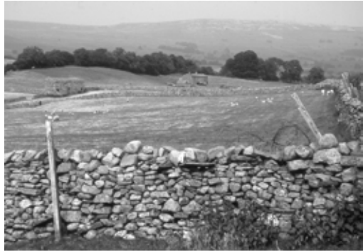
Figure 24. A common sight in the countryside of England was the abundance of dry stone fences that are constructed without mortar, but are very stable. Photo by R. Wayne Campbell.
