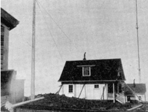
Figure 312. View of the lighthouse wireless buildings on Triangle Island in about 1915. Note the support timbers needed to brace the building against ferocious winds. Photo by T.E. Morrison, Agent, Department of Transport, Victoria, BC, courtesy G. Clifford Carl.
