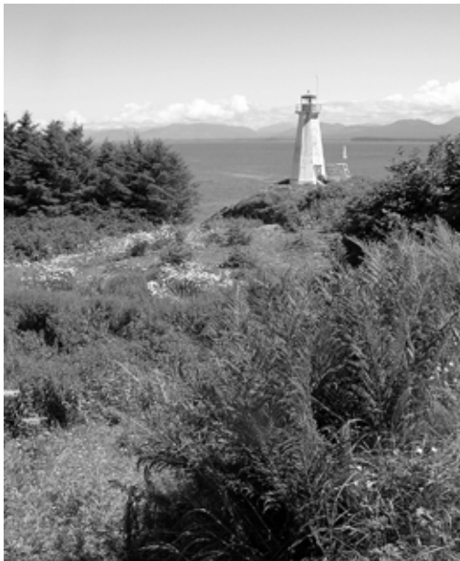
Figure 33. Lucy Islands lighthouse stands on the eastern point of the largest islet in the Lucy Islands group in Chatham Sound. From 1906 until 1988 it was a manned station, but now only the automated light tower remains. Photo by Moira J.F. Lemon, 18 July 2006.
